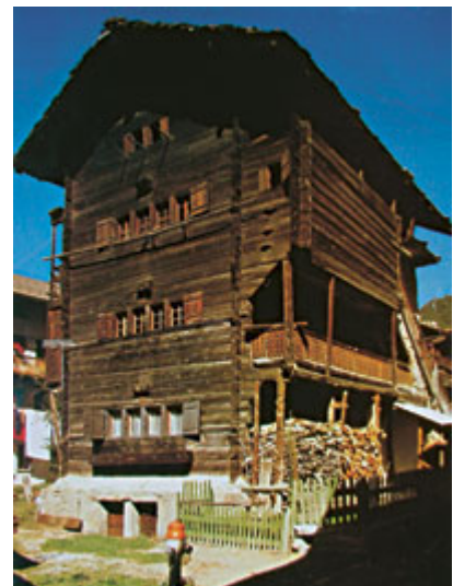
Fig. 2: A typical log construction building
