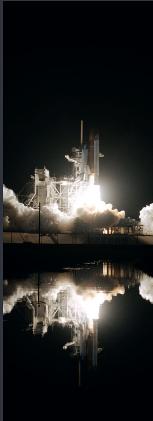
Launch facilities and services
